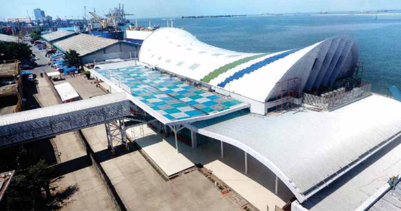
Proyek atap berlapis enamel (Terminal penumpang Pelindo IV) Enameled Roof Project (Pelindo IV Passenger)
